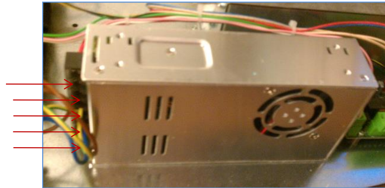
Remove electrical wires
